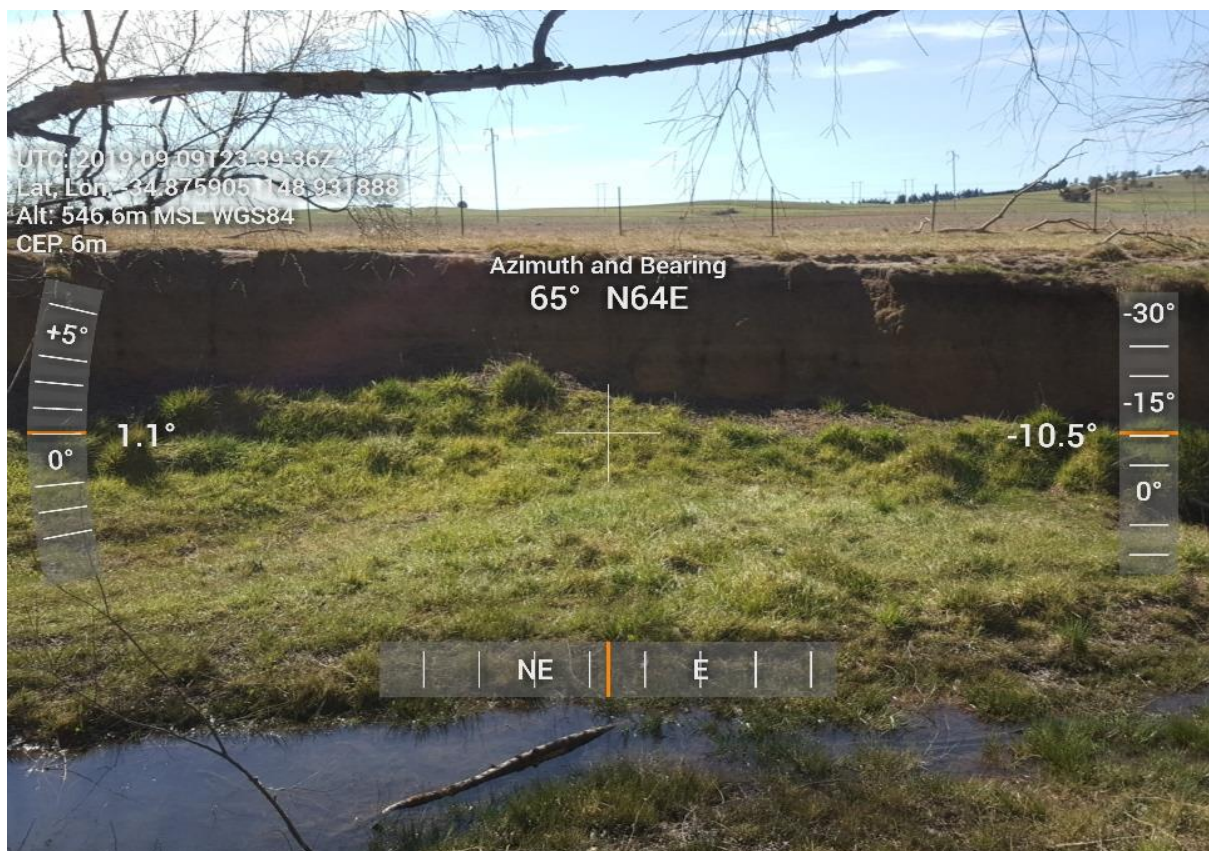
Figure 10: Section of stabilised creekbank erosion
